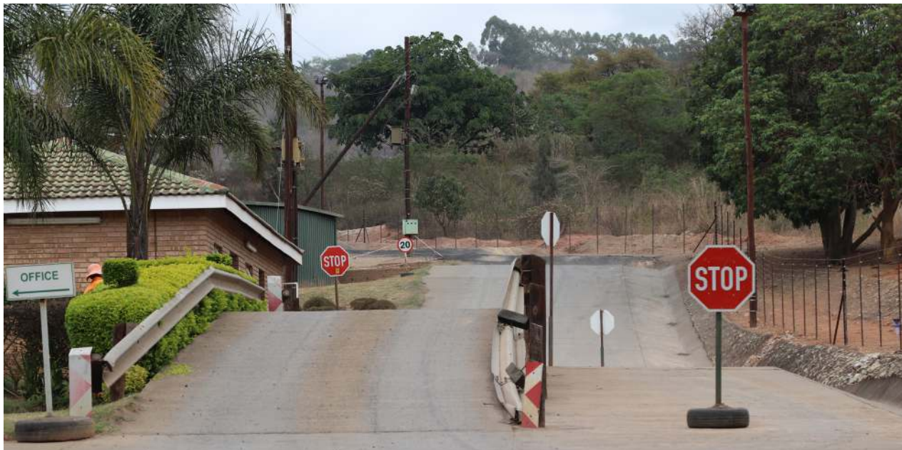
A successful landfill site in Tzaneen, with an operative weighbridge, fence and complete infrastructure
