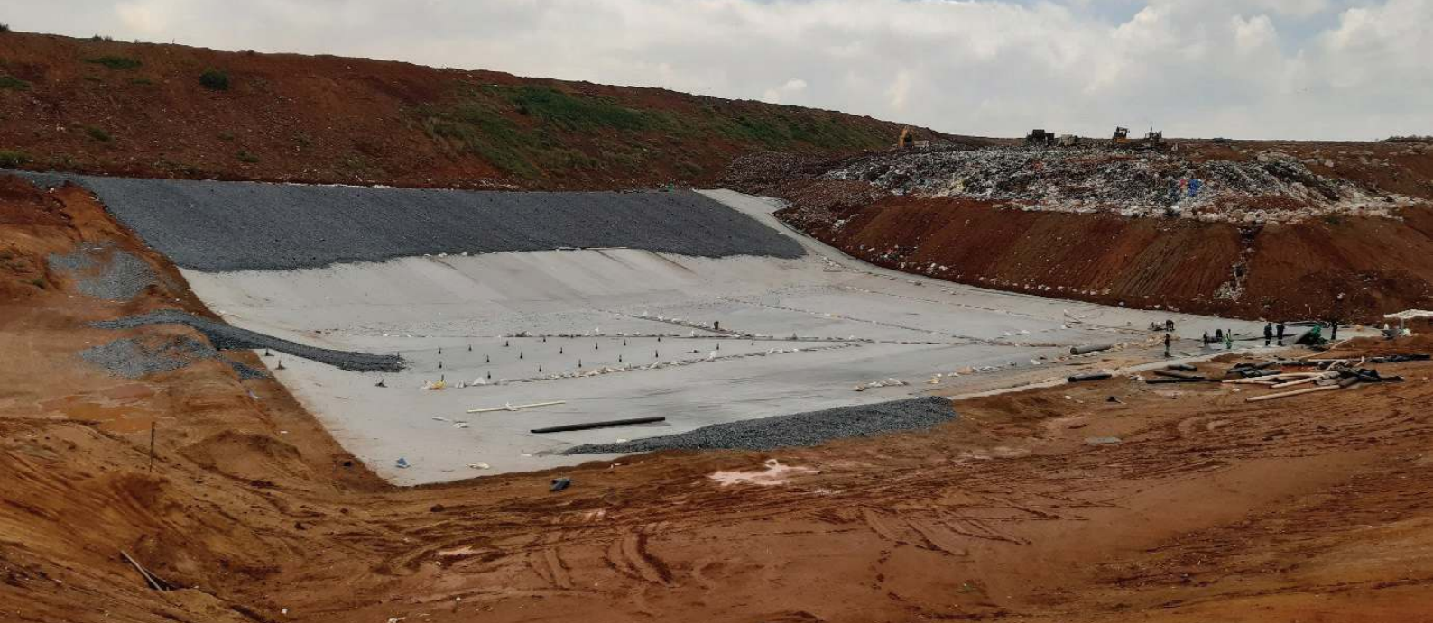
The Waste Group Class B liner being completed at the Mooiplaas landfill site in Centurion, Gauteng
