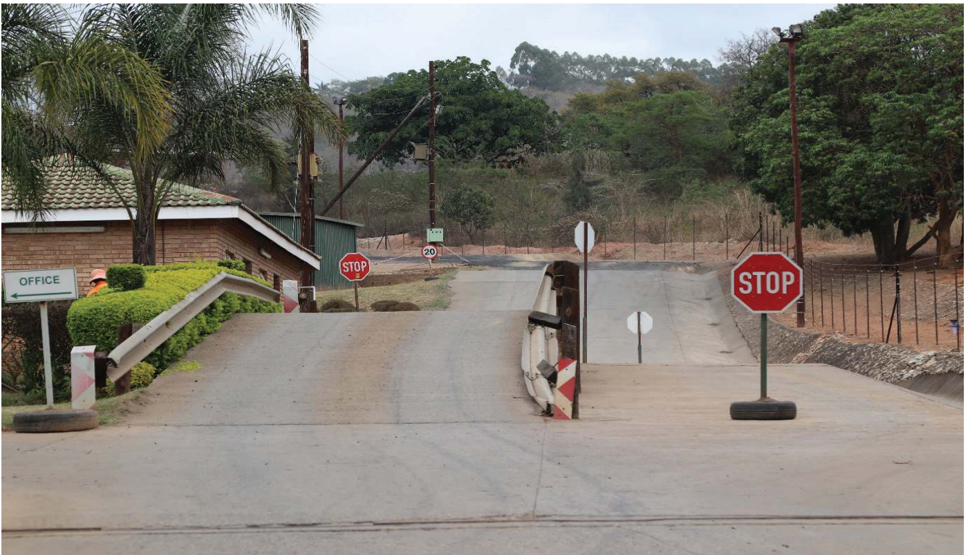
An impeccable landfill site in Tzaneen, with an operative weighbridge, fence and complete infrastructure
