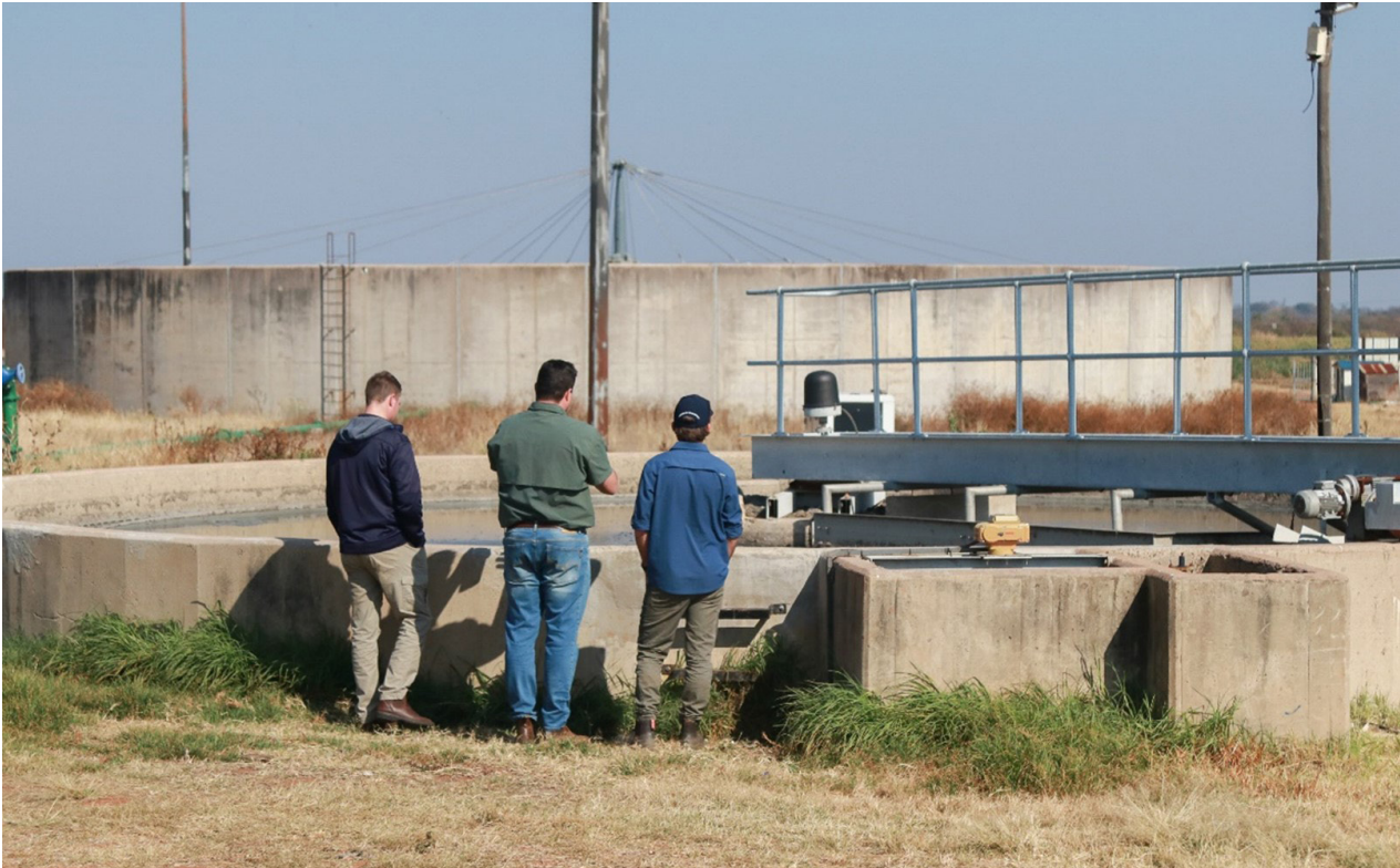
Figure 7: Warmbad's SWWTW during AfriForum's green drop visit for 2023
