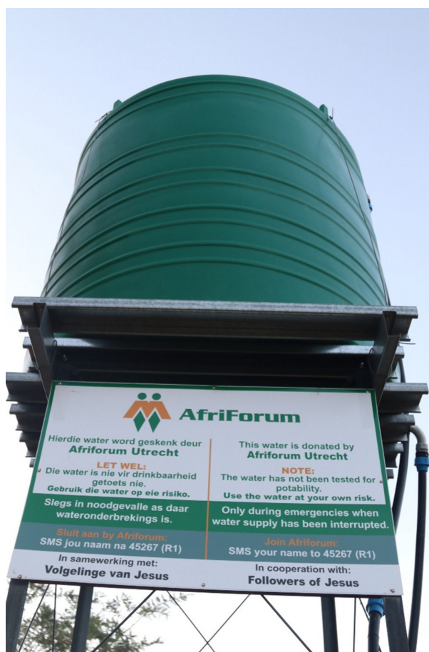
Figure 1: An emergency water point set up by an AfriForum branch
